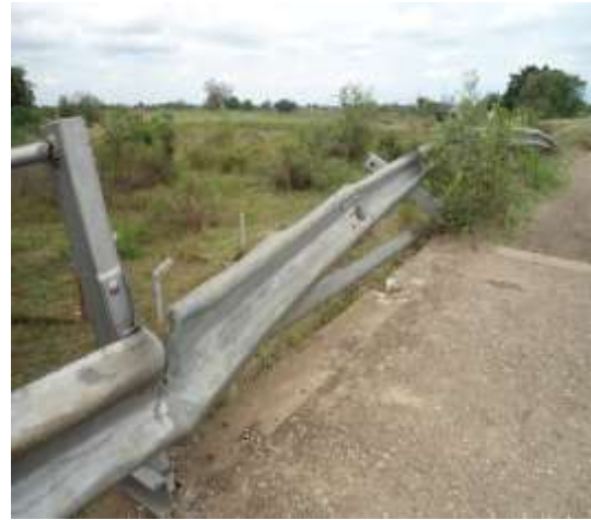
Figure 4.5 Traffic Impact within the Parapet
